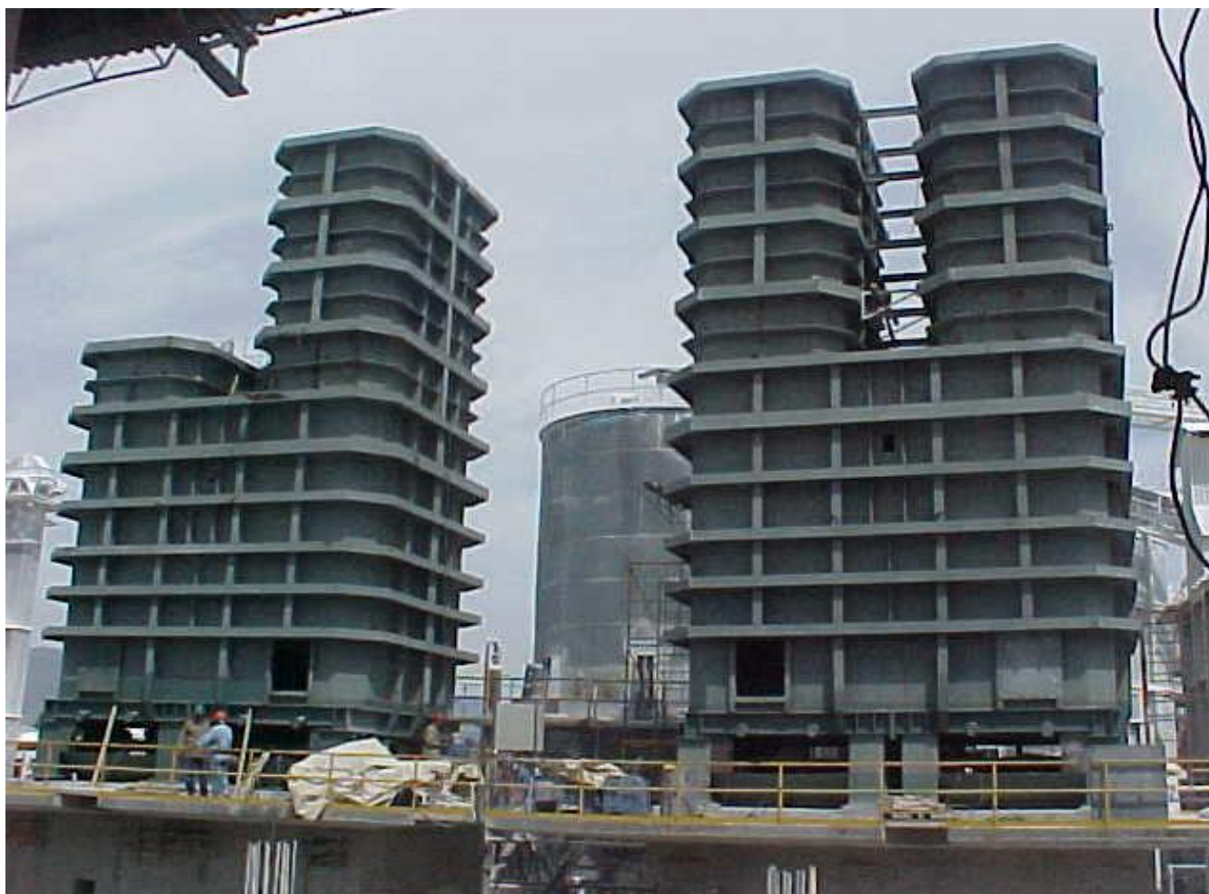
HORNOS MAERZ CALERAS APASCO, HIDALGO
